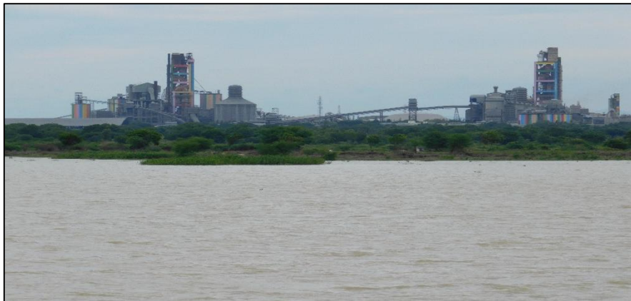
Lake restoration, Dalmiapuram Plant
