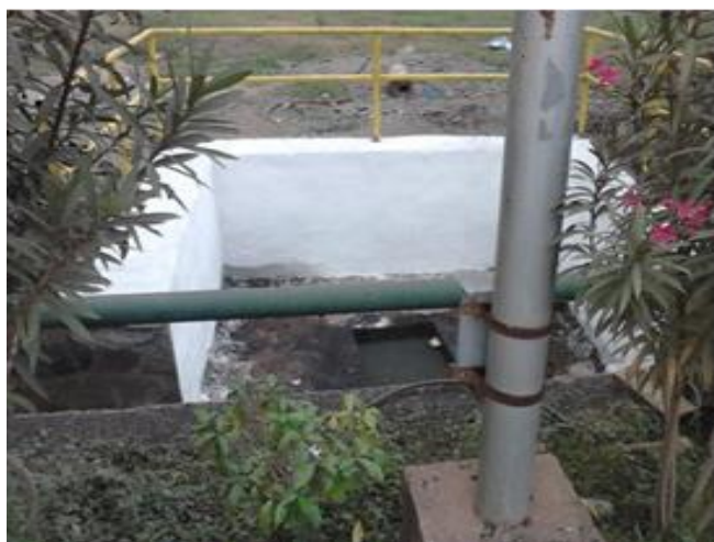
Drain Water Harvesting Pit
