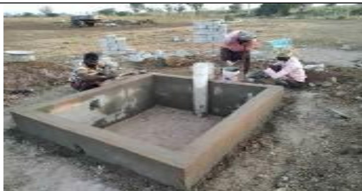
Bore well Recharge structure work in progress at Bheemagundam village watershed area
