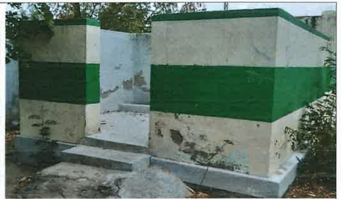
Sanitation Complex (Before)
