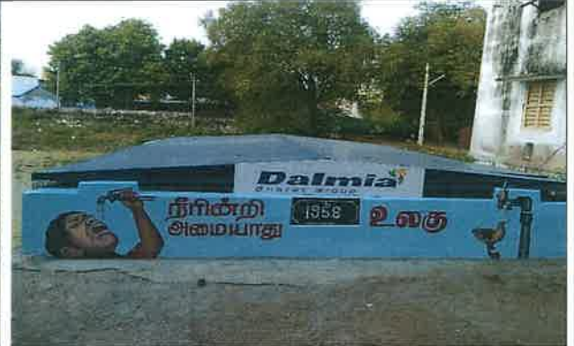
Mechanical Shed and Metal door to well (After)
