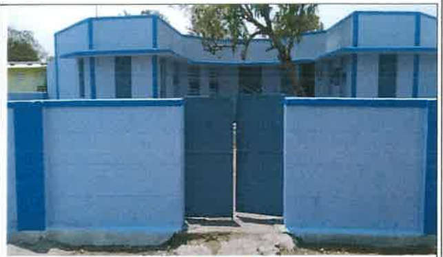
Anganwadi Samathuvapuram (After)
