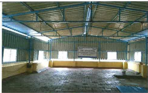
DSP office Shed (After)
