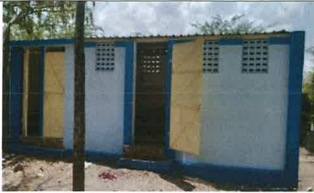
Uppathur School Sanitation Block (Before)
