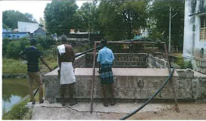
Shed and Metal door Closer to Well (Before)
