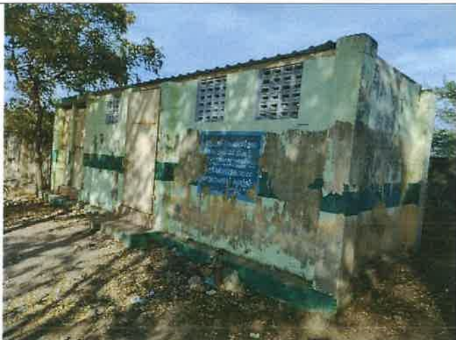
Govt Hr. School Sanitation block (Before)
