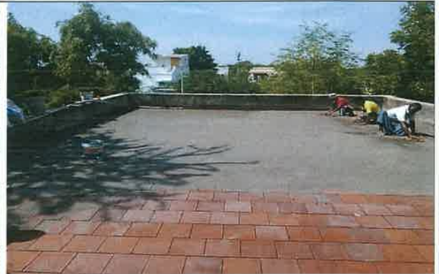
Weathering water proof tile laying work (After)
