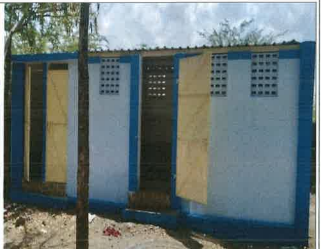
Govt. Hr. School Sanitation block (After)
