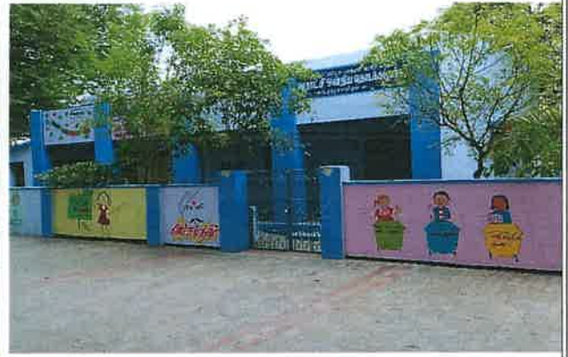
P.U. Primary school at Muthusampuram (After)
