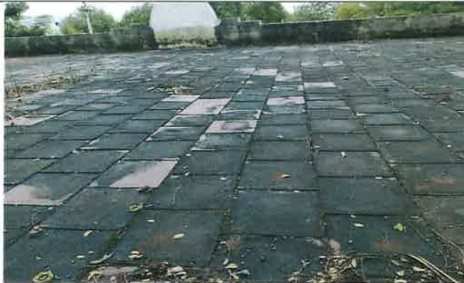
Weathering water proof tile laying work (Before)
