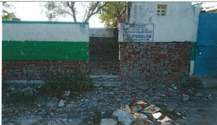
Sanitation Complex (Before)
