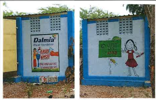
Uppathur School Sanitation Block (After)
