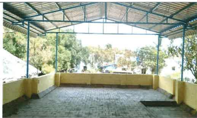
DSP office Shed (Before)
